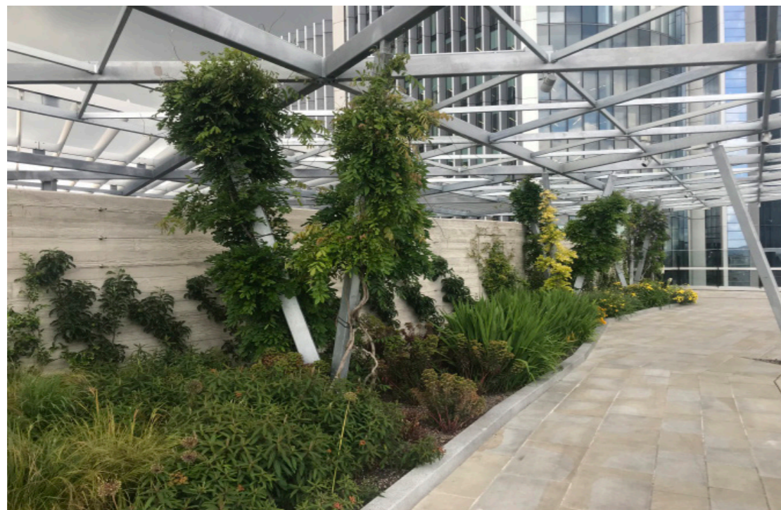
Figure 5. Roof gardens are an effective source control element in sustainable drainage systems
